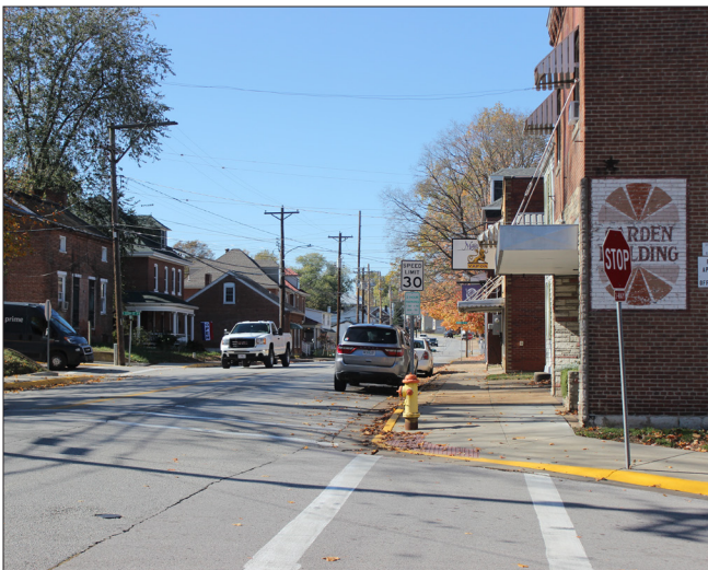
W. 5 TH STREET MIXED-USE BUILDINGS
