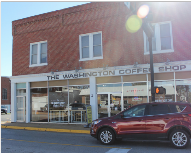
W. 5 TH STREET SIDEWALK AND TRADITIONAL STOREFRONT
