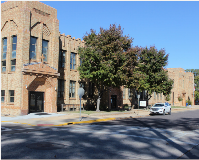
ST. FRANCIS BORGIA ELEMENTARY SCHOOL
