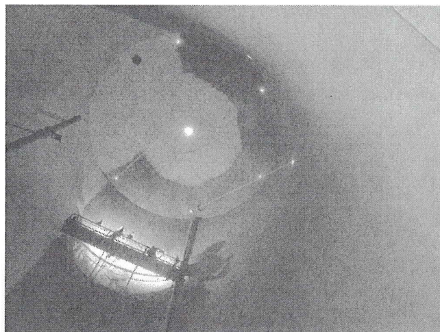
Interior Tank – Blasting
