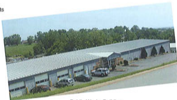
Public Works Building
