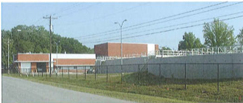
New Wastewater Treatment Plant - 2009
